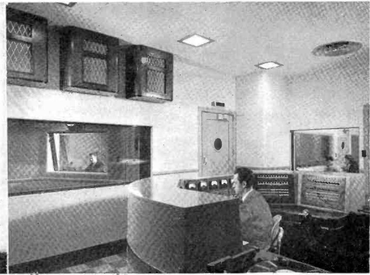
MASTER CONTROL ROOM , center of technical operations. It handles switching functions of six studios. Operator can see into three studios.
